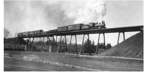
Railway bridge across the Conestoga River, looking west
