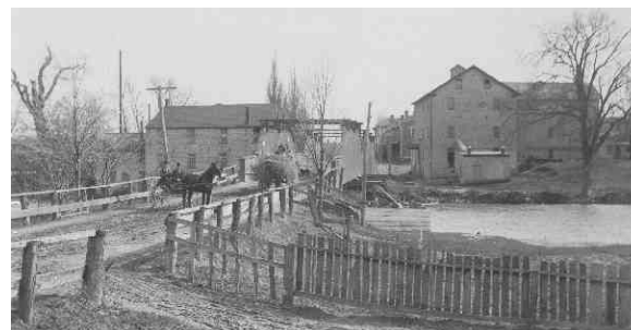
Bridge across the Conestoga River, looking south
